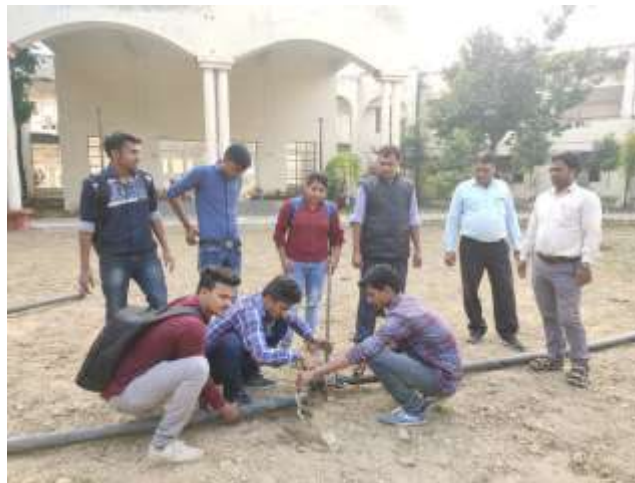
Fig. A view of installation of sprinkler irrigation system
