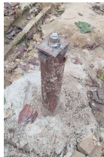
c) 4-inch Boring
