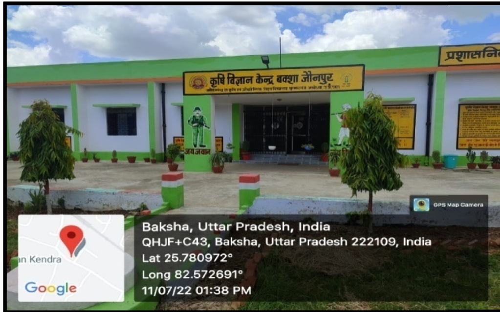
Administrative Building of KVK, Baksa, Jaunpur
