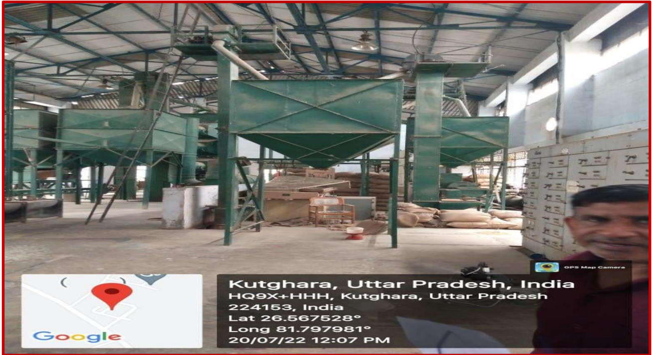
Seed Processing Plant
